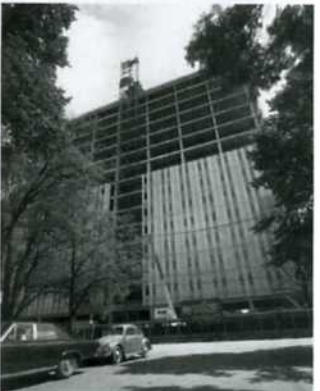
TUPPER MEDICAL BUILDING, COLLEGE STREET (below: during construction in 1967).
